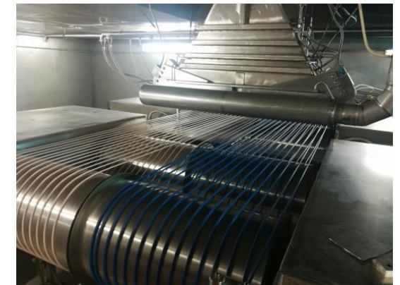
2 In & 2 Out wires treatment by one ELV accelerator in JSC "Electrocable Works, Kolchugino" Speed of each line – 400 m/min
